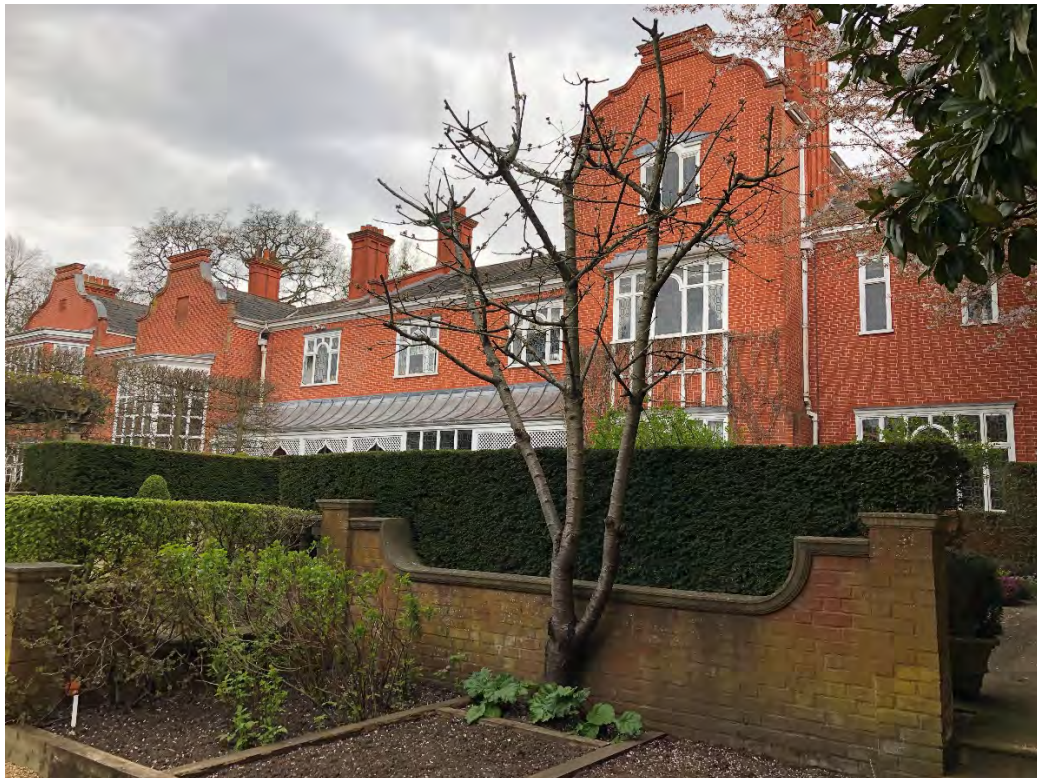
The last bay defines the Northern end of the house, where the extension built in 1998 now houses the kitchen, at ground level.
