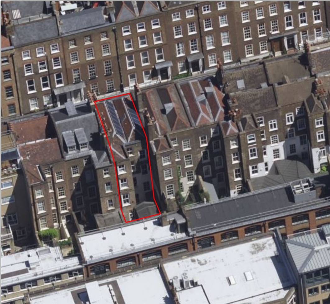
Figure 1 - Aerial photo of the Site and neighbouring buildings (© Bing)
