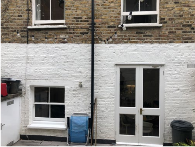
fig.4. Existing rear view of the timber window & double doors
