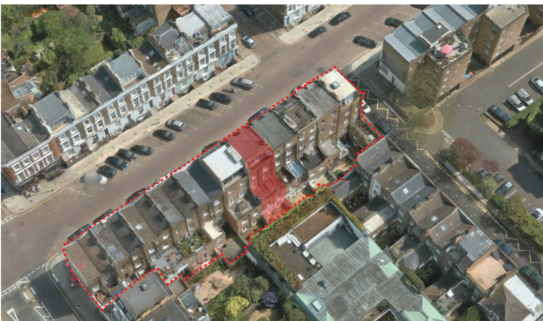
fig. 3. Aerial view showing the rear of the terrace of houses nos. 50-40 Chalcot Road
