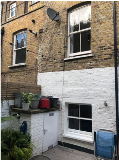
fig.5. View from the garden showing the existing window
