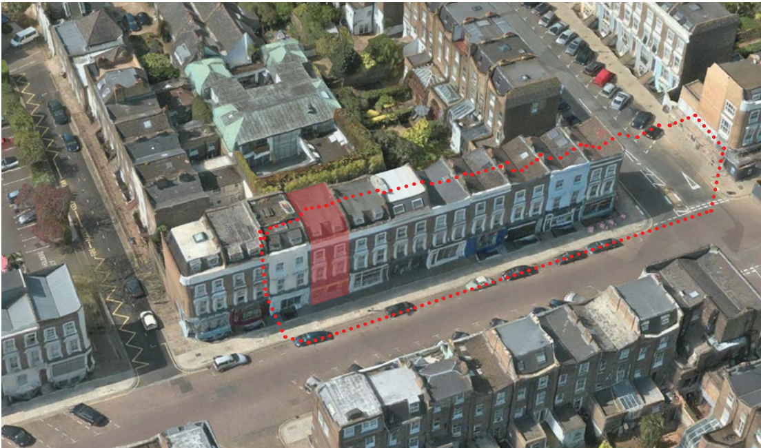
fig. 2. Aerial view showing the terrace of houses nos. 50-40 Chalcot Road
