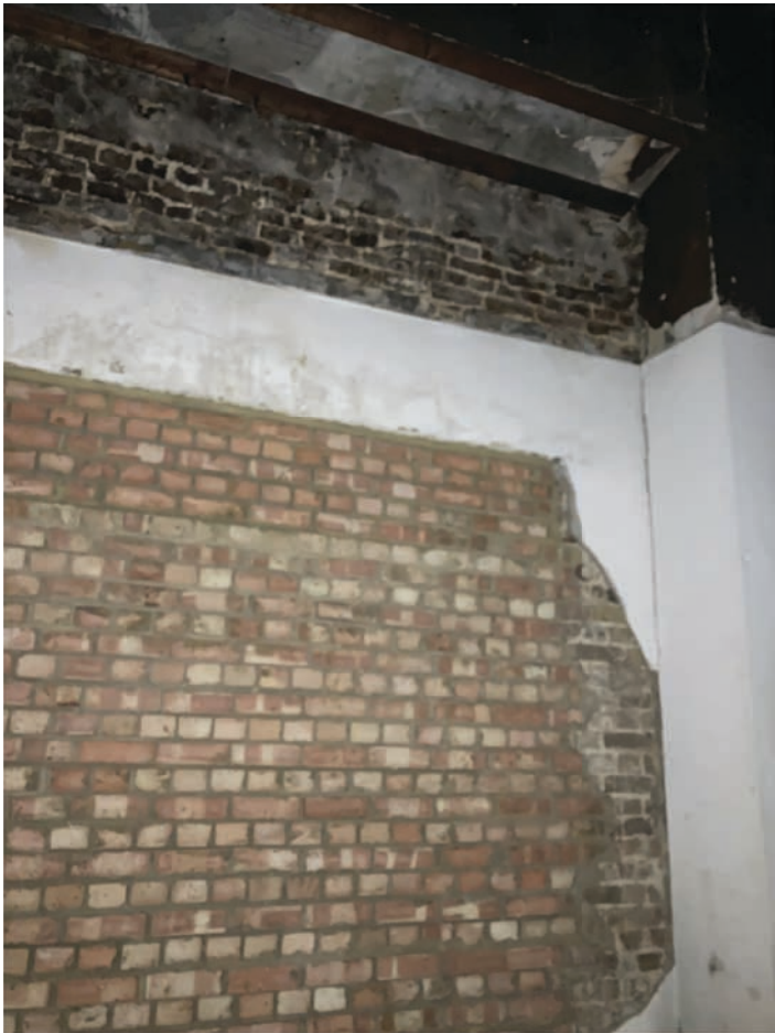
Internal face of the Prince of Wales elevation showing blocked up opening (formed 1960, bricked up 1984)
