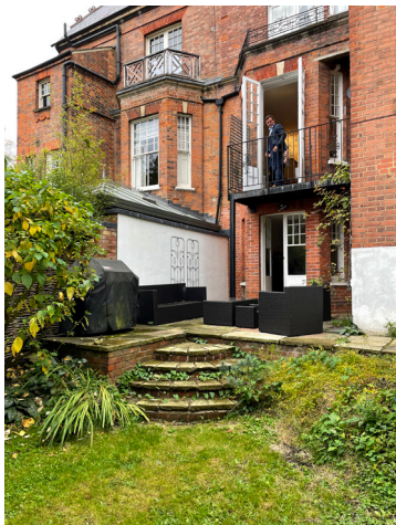
Rear elevation and existing lower ground floor rear extension to neighbouring property no.6 Well Road
