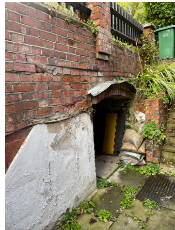
Side passage and store below front path
