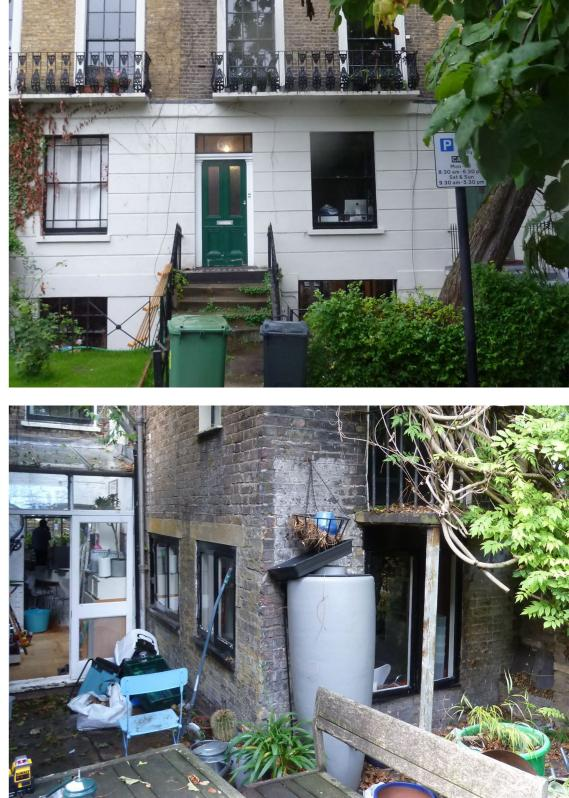
Rear outrigger from garden Outrigger in very poor condition and overgrown Rake out and re-point mortar - see GA201. New staircase and wall built out to support replacement landing see GA201.
