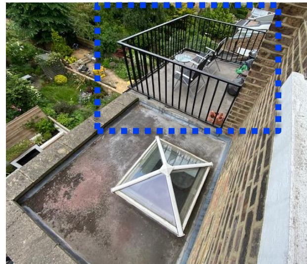
Accessible terrace at No. 22
