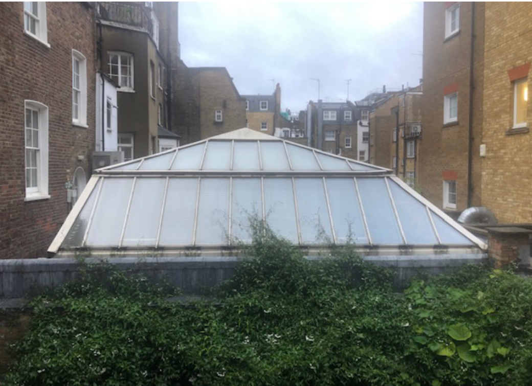
4. View of existing extension from No.29 Percy Street
