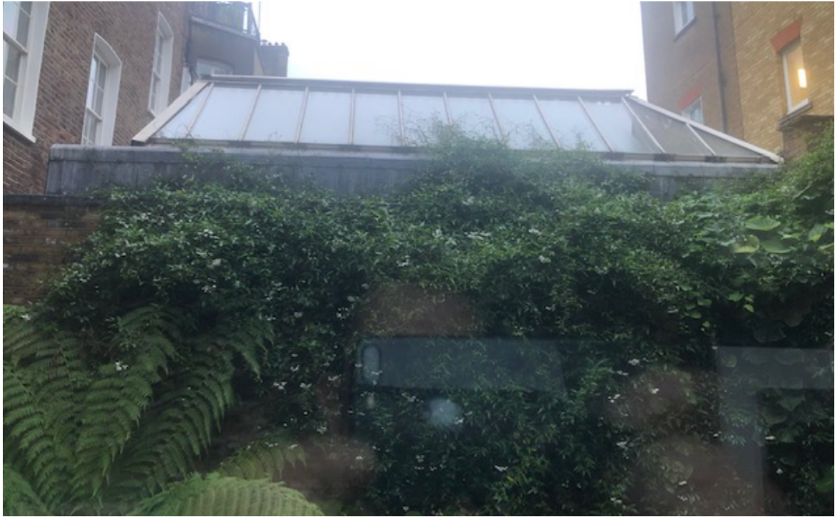
5. View of extension from rear garden of No.29
