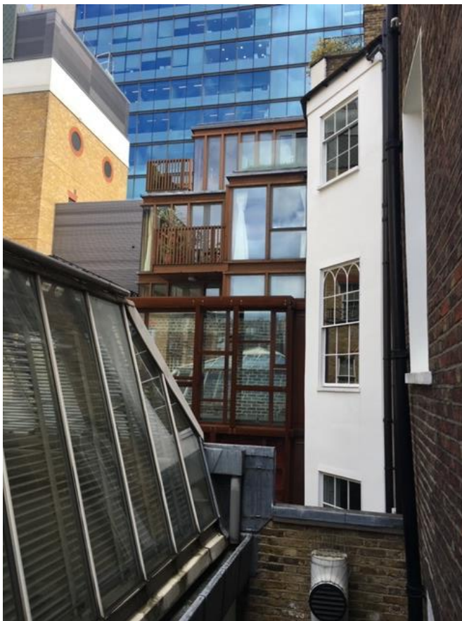
2. View east showing existing upper floor terraces at No.29 Percy Street
