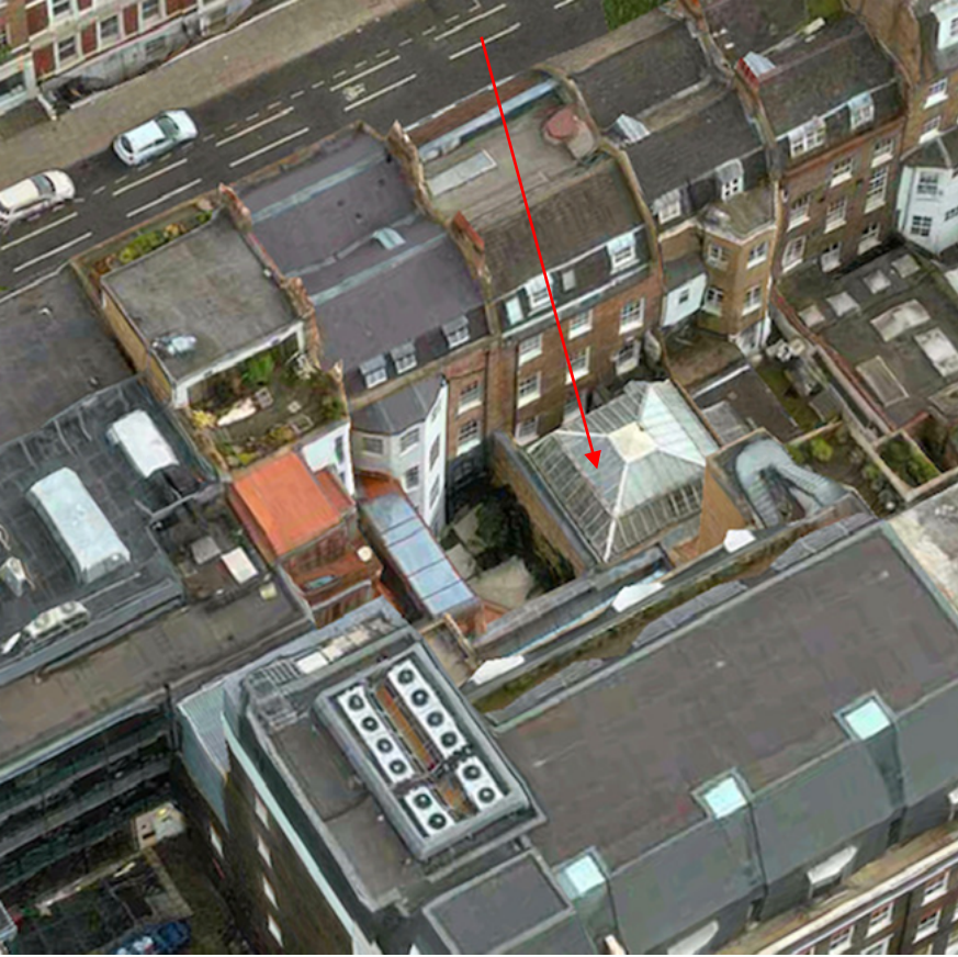
3. Aerial view showing existing rear extension
