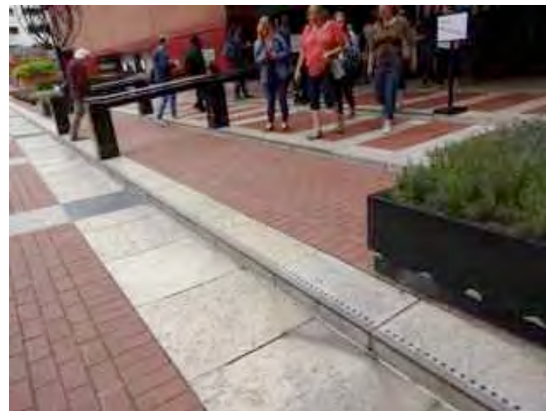
Existing shallow ramped single steps that are a trip hazard
