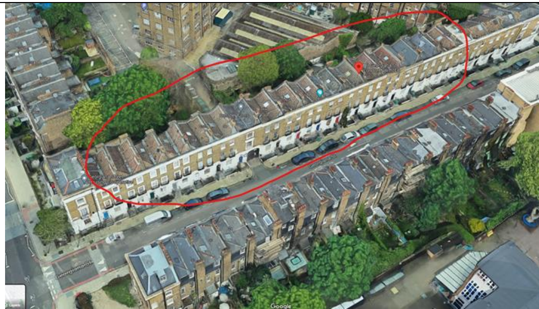
Aerial view of northern side of road showing 43 Georgiana St
