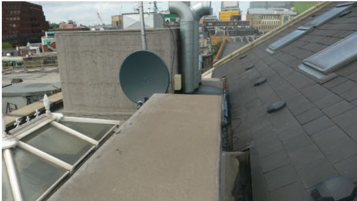
View from property the Cambridge Theatre to illustrate why a man-safe cable system is not practical as a solution to ensure safe maintenance working on the roof
