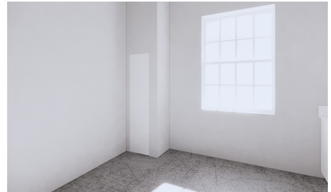
Above; Where size and shape of service enclosures has been adjusted new fire rated risers are to be formed. These will be finished to match the adjoining walls and have neat junctions to the existing fabric. Flush access doors will provide access.
