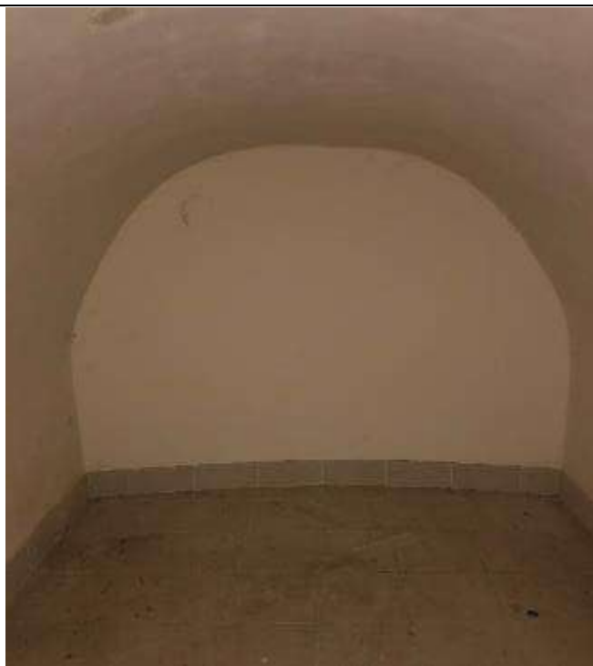
Barrel Vaulted areas under Footpath
