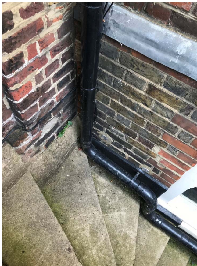
Figure 8 plastic rainwater pipe with Doulton tubes above
