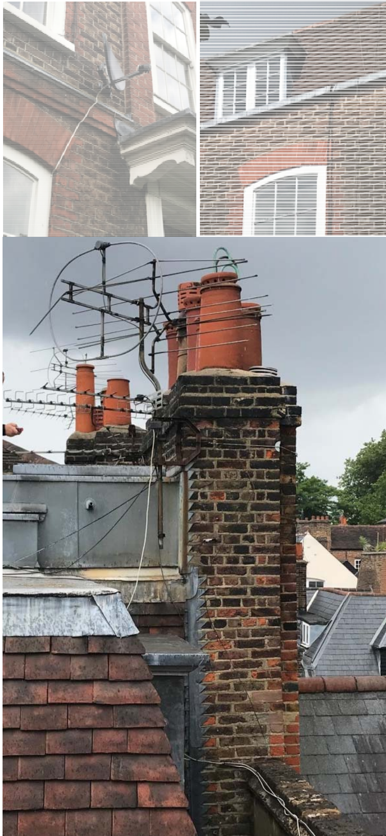
Figure 3 Typical surface mounted cabling on the outside of the building
