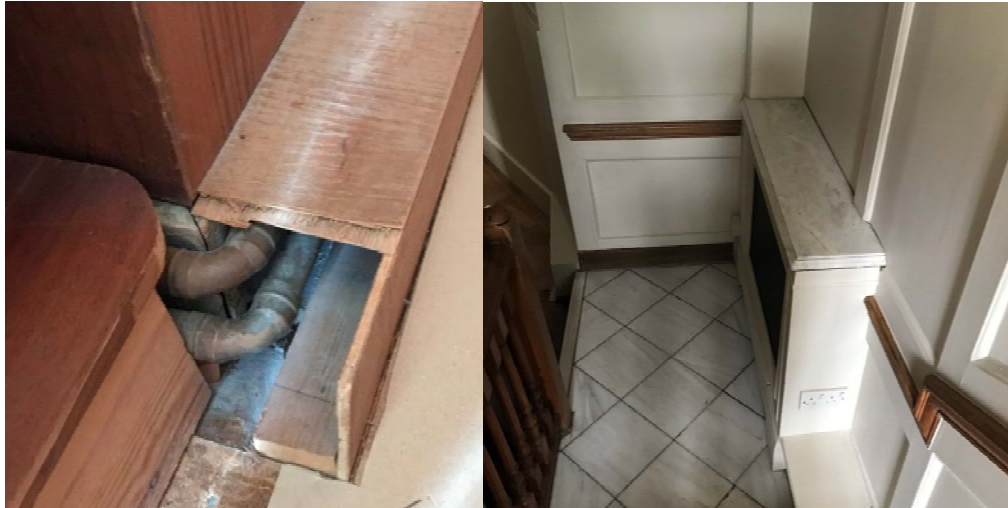
Figure 4: internal heating pipework and boxed in radiators on the main stairs
