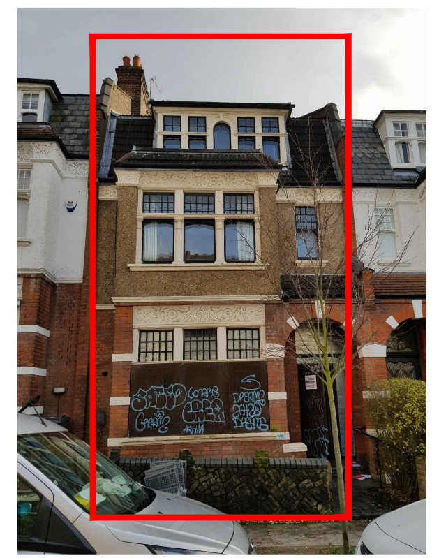
3 | EXISTING FRONT FACADE
