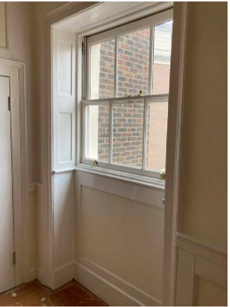
Figure 114, Top - A general view of the room, showing the fireplace mantle left in-situ. Figure 115, Middle - The windows retain much of their historic joinery, and the dado encircling the room is also historic. Figure 116, Bottom - Another view of the historic windows, with their historic joinery.
