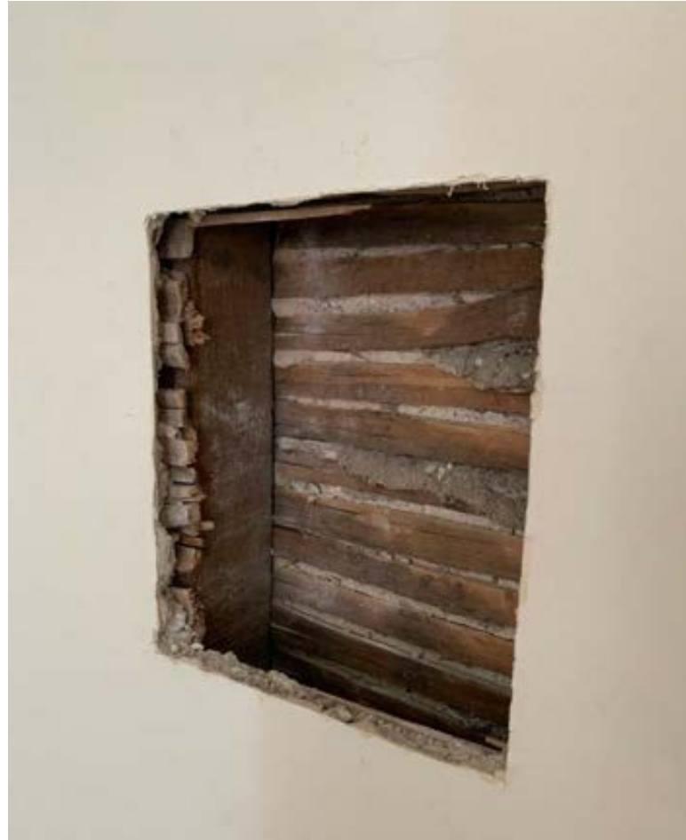
Figure 39. View B - Existing Lath and Plaster
