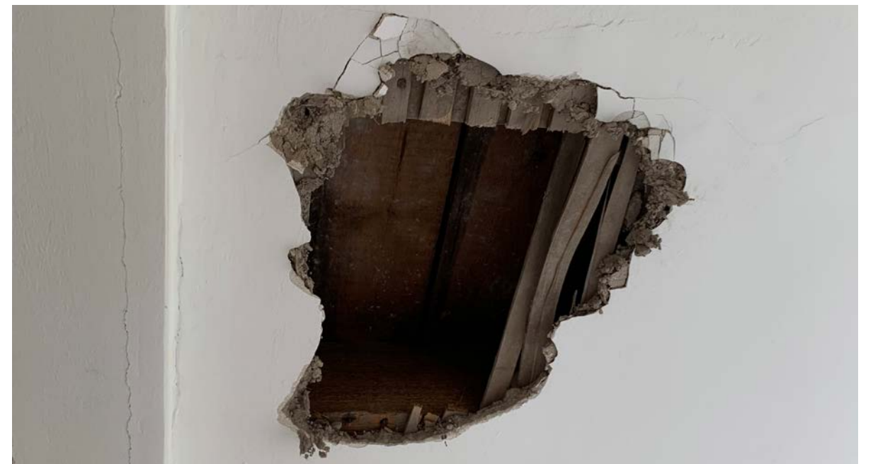
Figure 63. View A - View of historic lath and plaster
