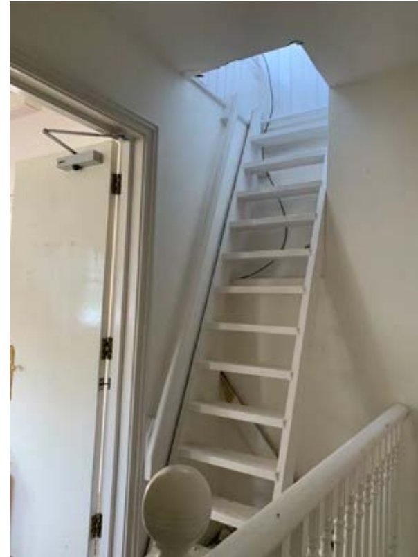
Figure 14. Ladder stair to existing escape window on fourth floor.
