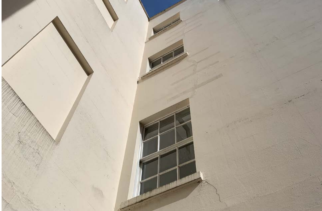
Figure 3. Existing photo of no. 19 Southampton Place viewed from Barter Street showing condition of render.
