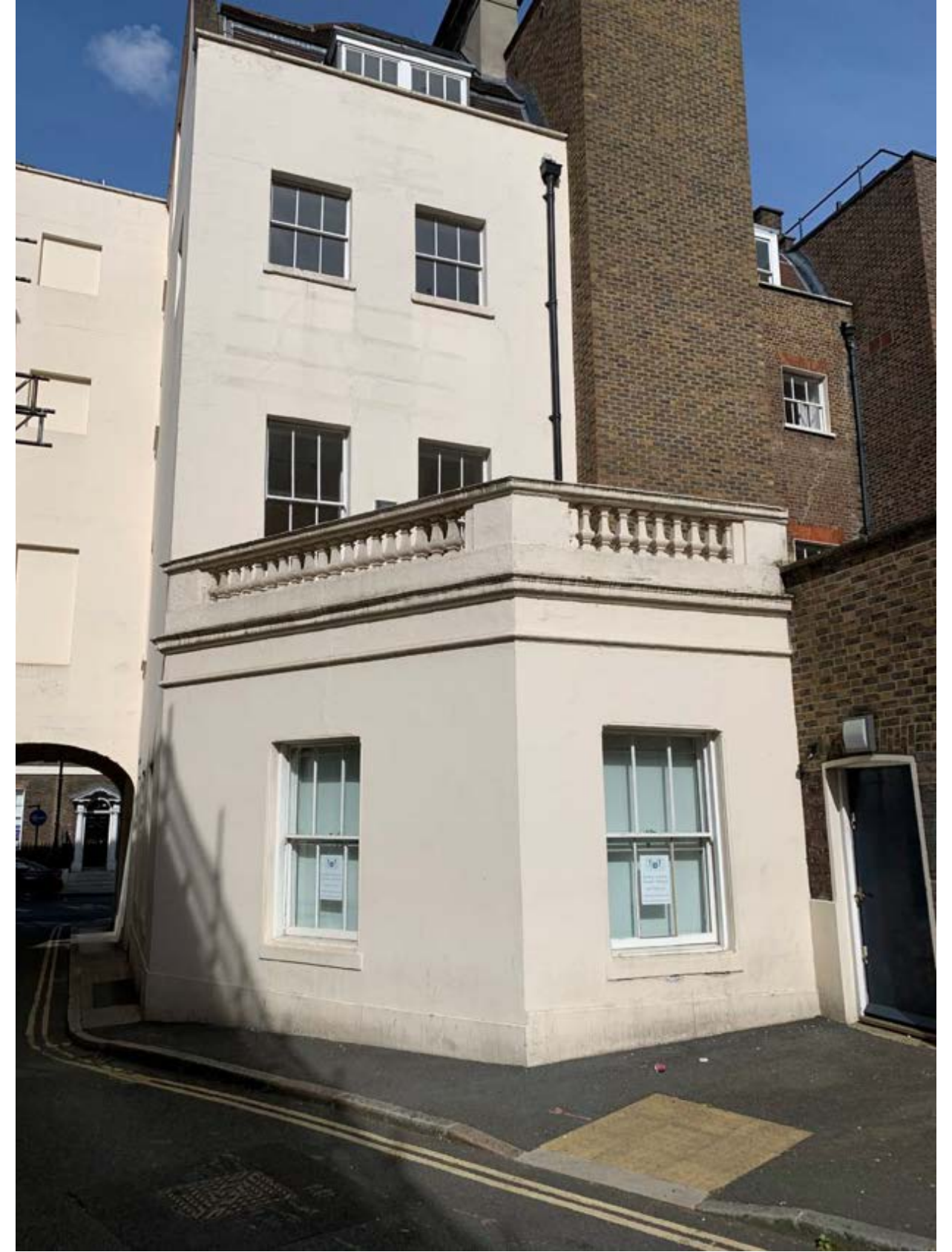
Figure 5. Rear of 18 & 19 Southampton Place showing facade condition and 1970s lift and WC core.
