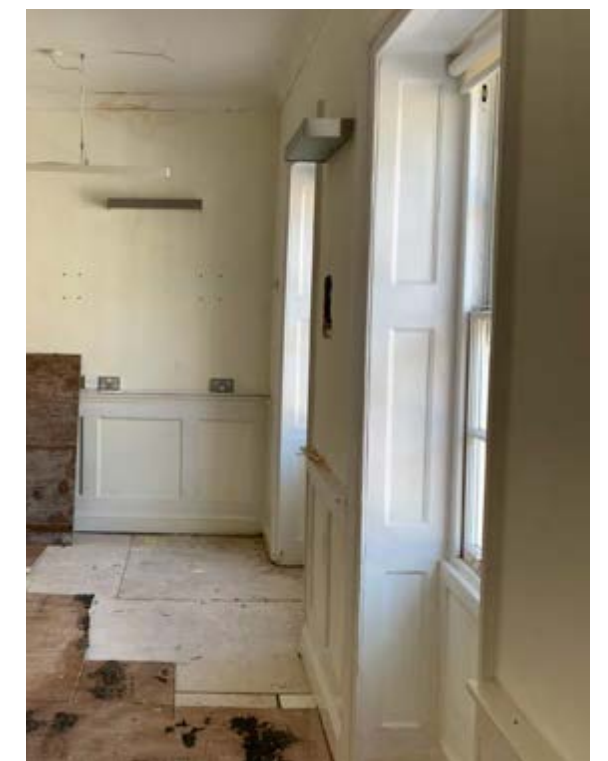
Figure 56. View F- View of historic timber panelling around window reveals.
