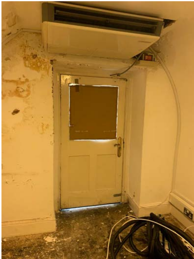
Figure 35. View A - Existing external door and broken glazing
