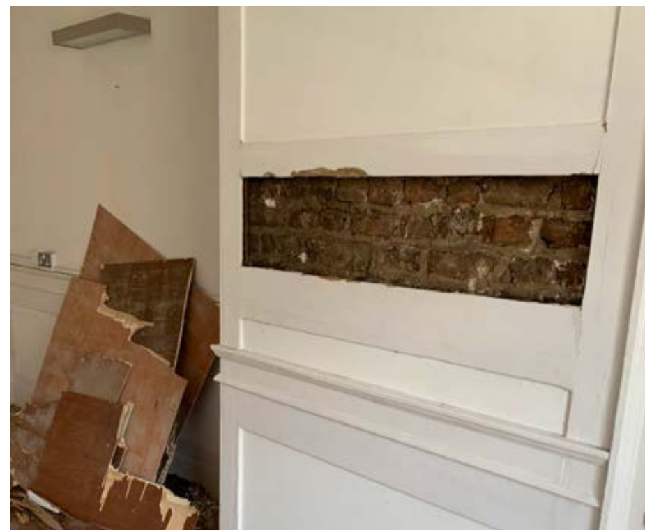
Figure 55. View E - View of missing timber panelling showing historic brickwork behind
