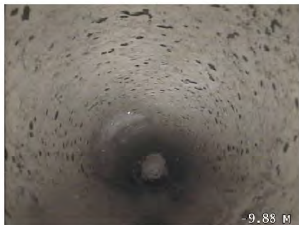
Start node type: Manhole
