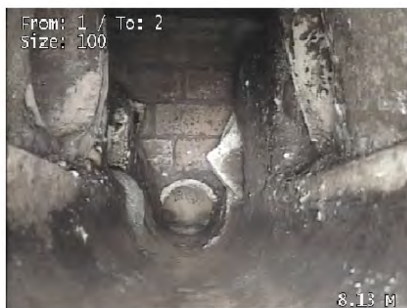
Finish node type, manhole, reference number 2
