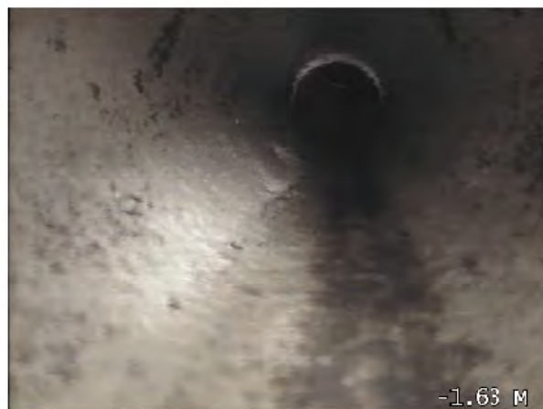
Start node type: Manhole
