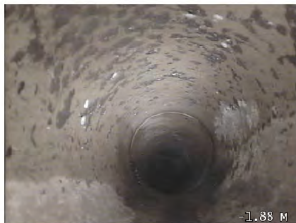
Start node type: Manhole
