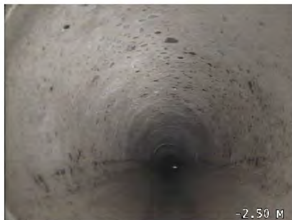
Start node type: Manhole
