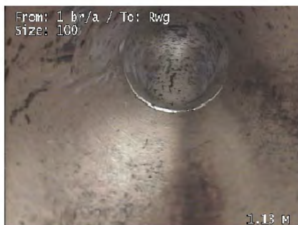
Line of drain/sewer deviates up half
