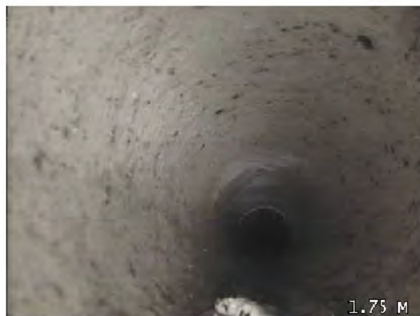
Start node type: Manhole
