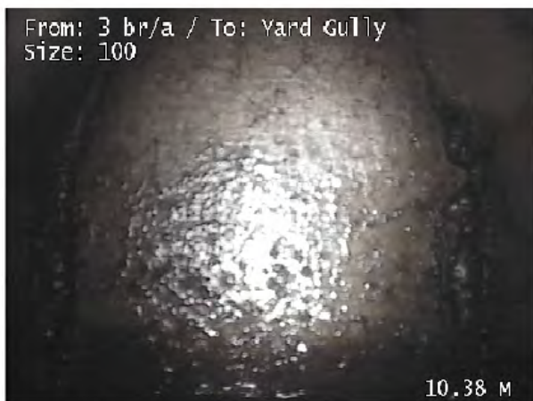
Yard gully Reached
