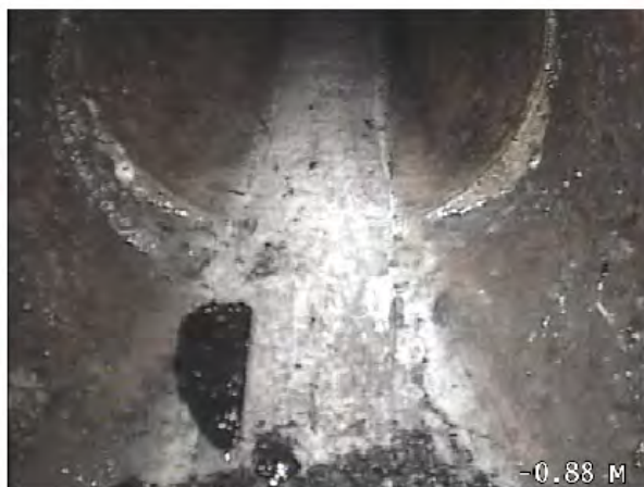
Start node type: Manhole
