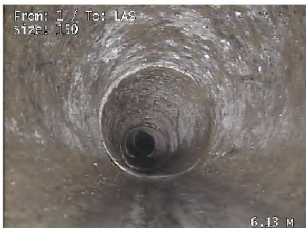
At boundary approx sewer depth 2.5
