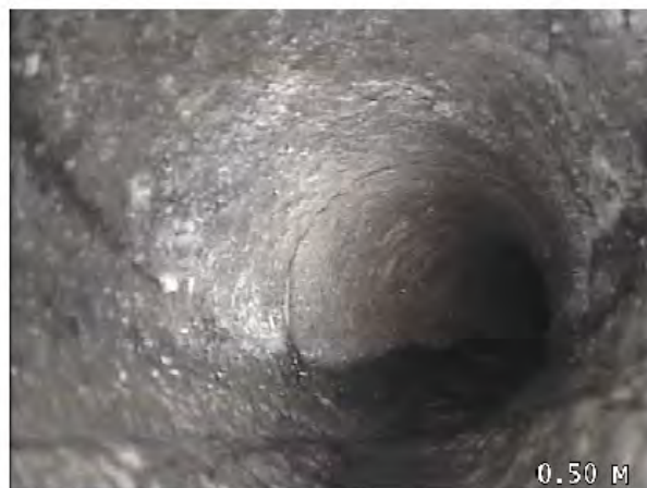
Start node type: Manhole
