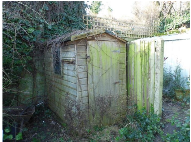
Plate 3: Timber shed to rear of property
