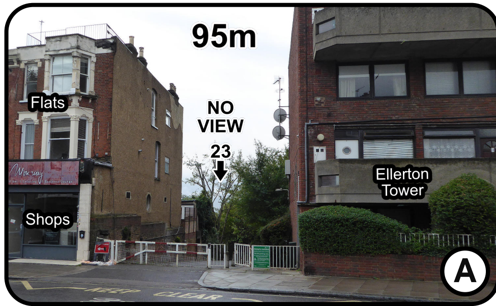
Gap beside Ellerton Tower on Mill Lane.
