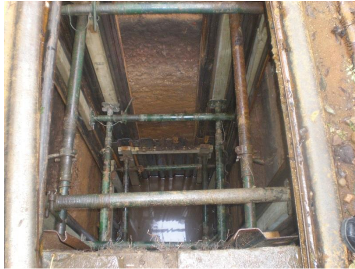
Figure 2 Propping
