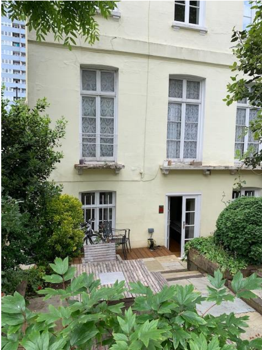
Image 5 (above): View from the garden looking at the rear elevation of 39 Priory Terrace. Rear facing East.
