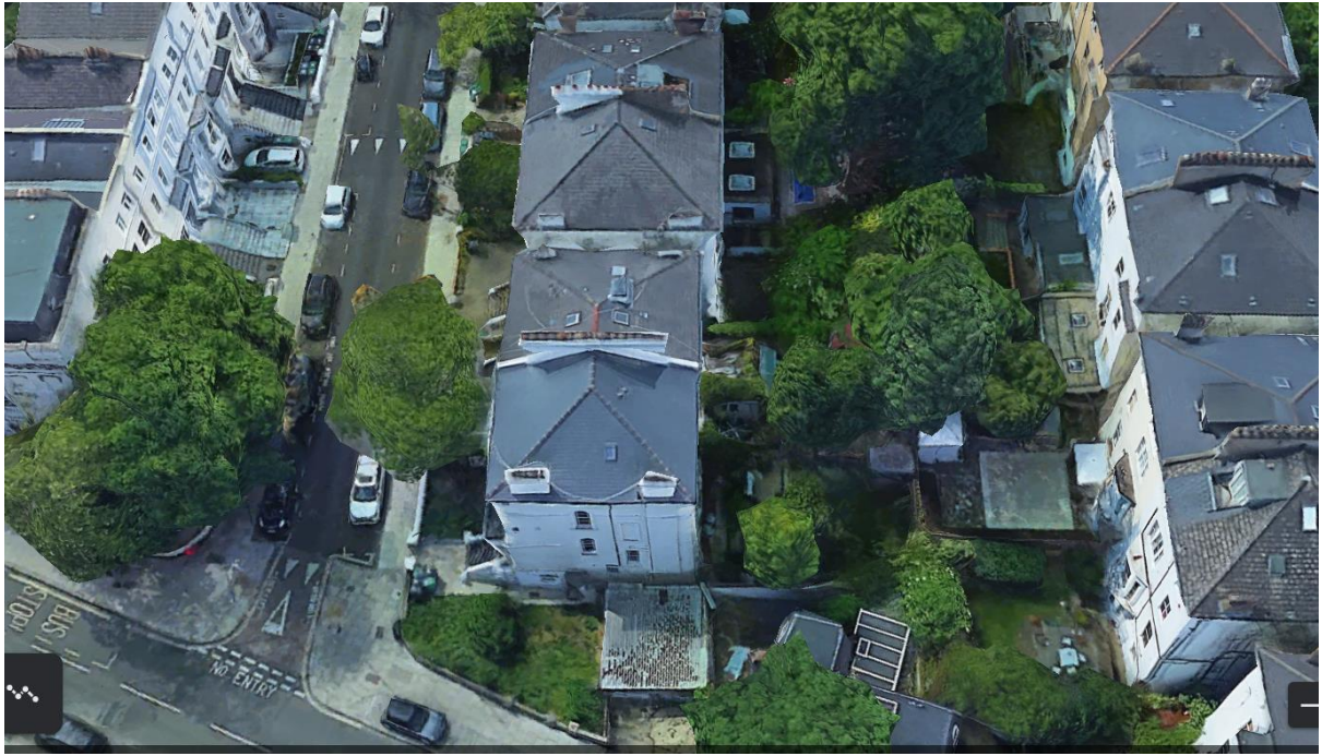
Image 1 (above): Aerial view of the site
