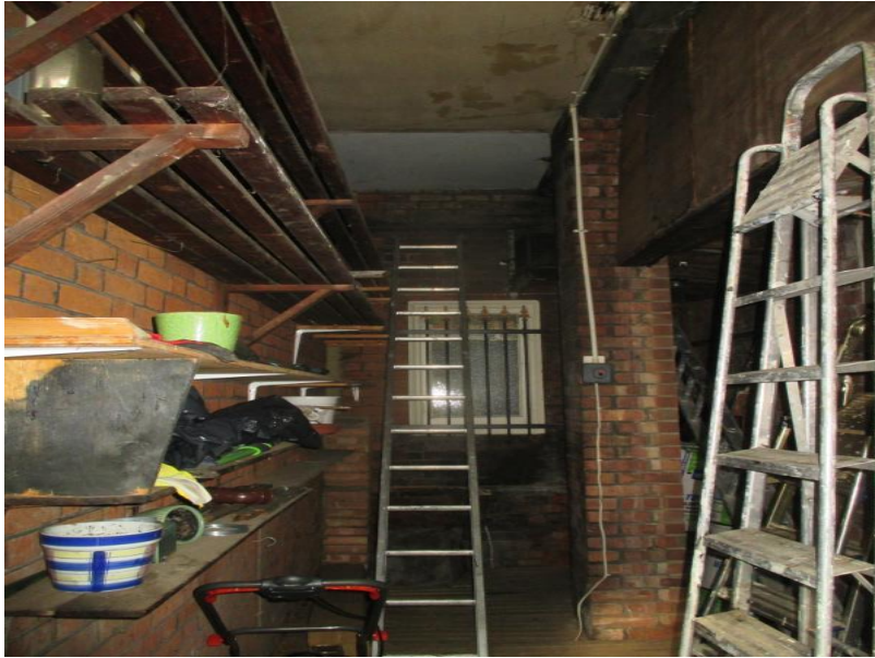
Inside of store room
