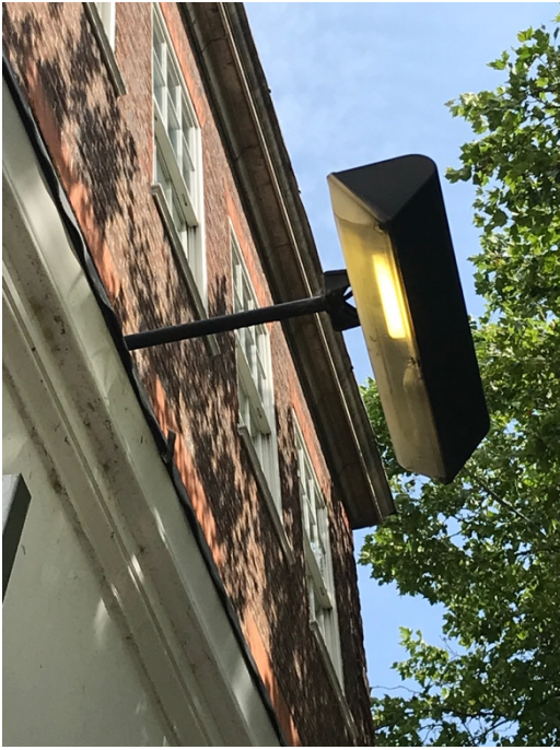
09: Existing Fascia Lighting
