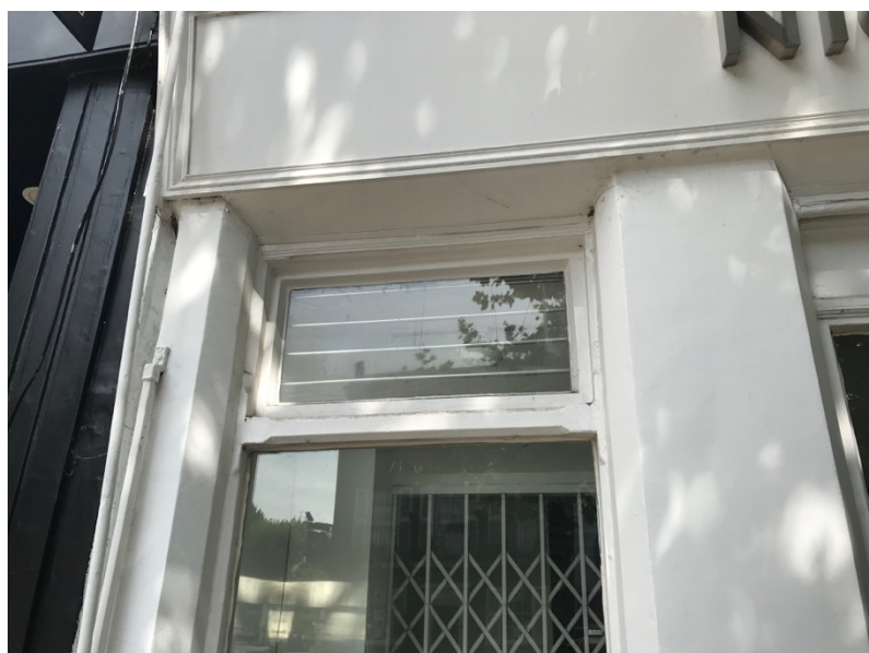
04: Existing Louvred Window
