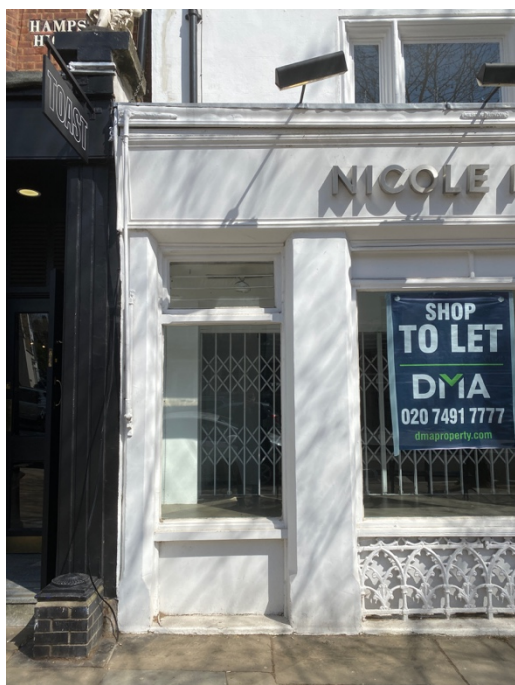
03: Existing Louvred Window
