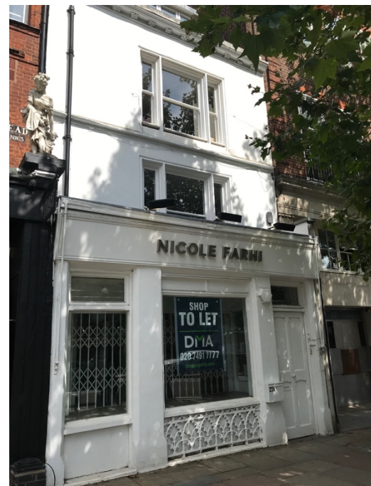
02: Shopfront Context Within Building
