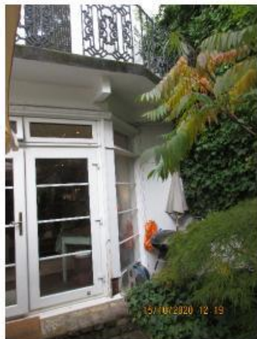
Balcony Pergola will sit underneath to train and control the massed vegetaion in the garden
