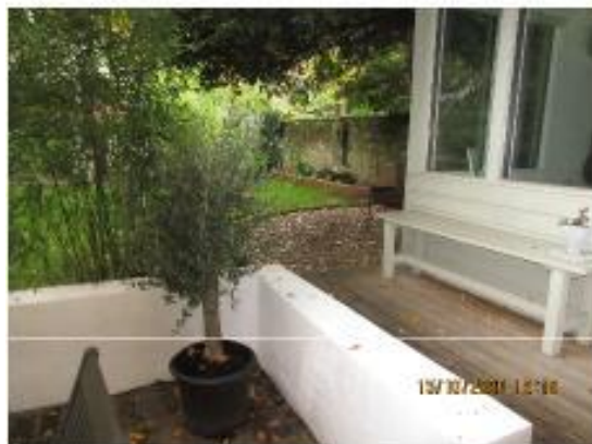
Dwarf walls existing form the base of the new pergola
