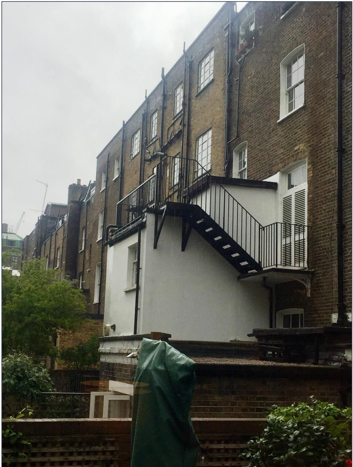
Fig 1. Western part of the rear elevation of Nos. 1–17 Regent Square. The white extension with roof terrace is at No. 8. The full-height external flue is at No. 13
