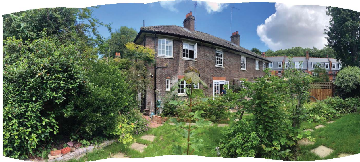
5. Overall view of garden and rear of building taken from the south western corner of the garden.
