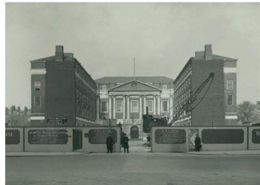
Figure 11: BMA house prior to the construction of the front wing.
