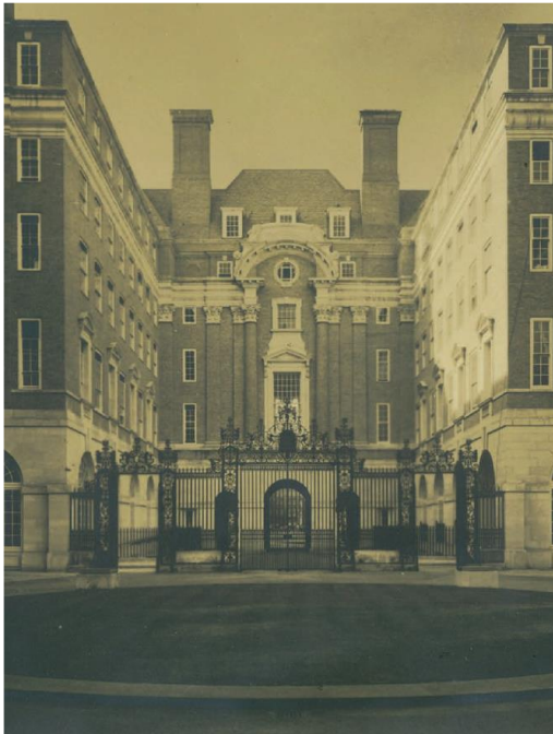
Figure 12: The courtyard prior to the construction of the memorial fountain.
