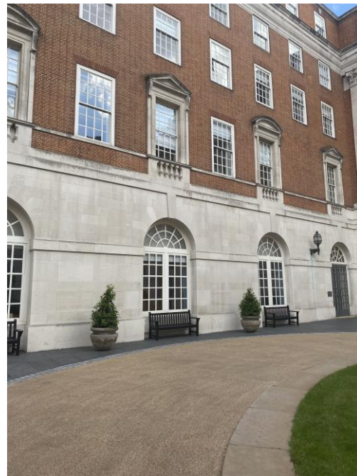
Figure 13: Existing courtyard finishes.
