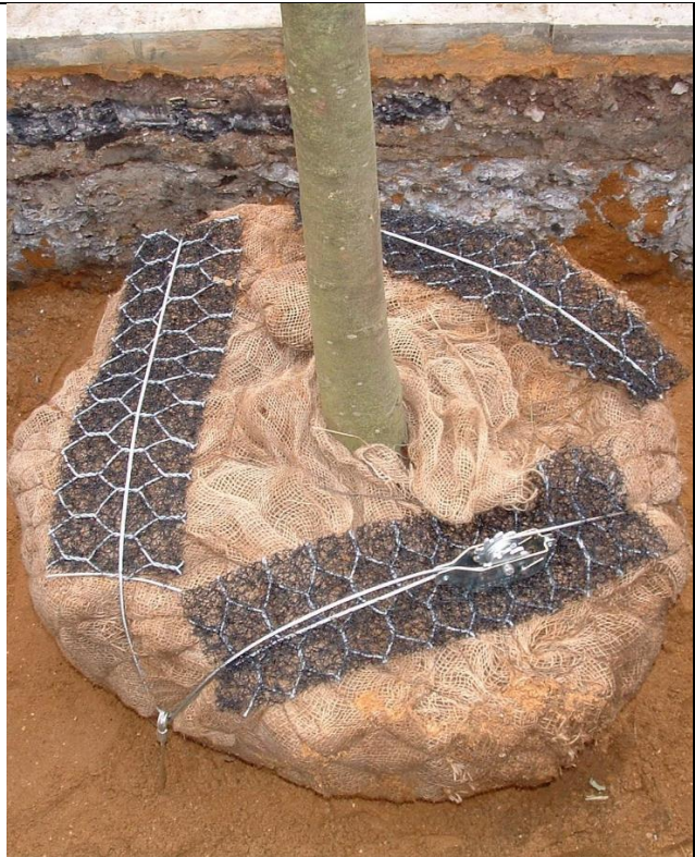
Example 5: Below ground cable anchor of tree
