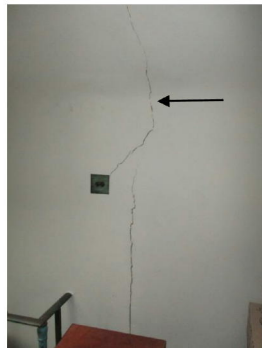
Cracking on rear addition junction in flat 6 rear bedroom
