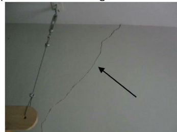
Cracking in flat 6 rear bedroom study room
