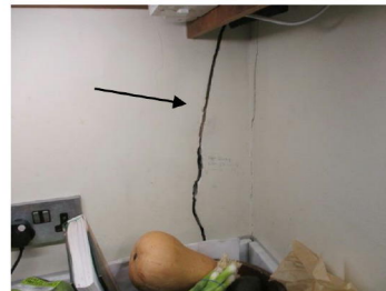
Cracking in flat 6 kitchen
