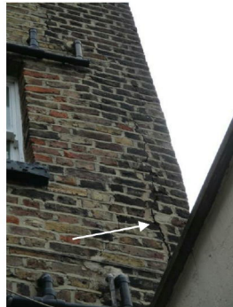
Cracking to rear elevation
