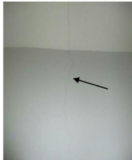
Unrelated cracking in flat 3 hall
