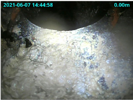
Fig 2.1: Line 1, pipework at higher level than channelling
