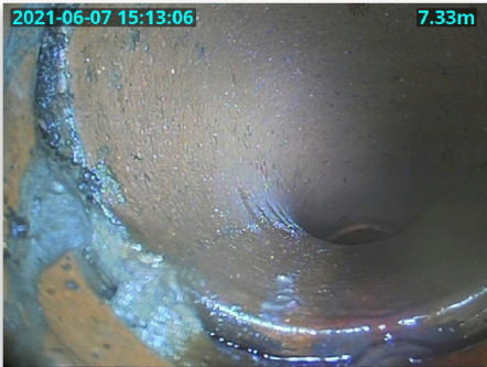
Fig 2.3: Line 2, joint displacement
