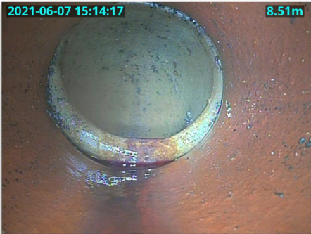
Fig 2.4: Line 2, joint displacement
