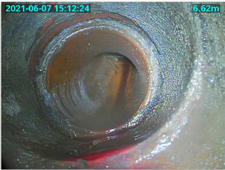
Fig 2.2: Line 2, joint displacement
