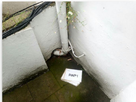
Fig 7.2: RWP1 that deviates off property then we believes loops around and connects into WG1
