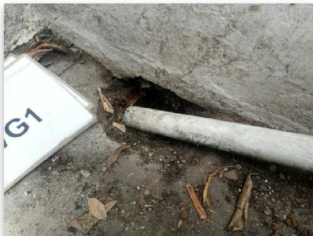
Fig 7.1: WG1, that is half recessed
