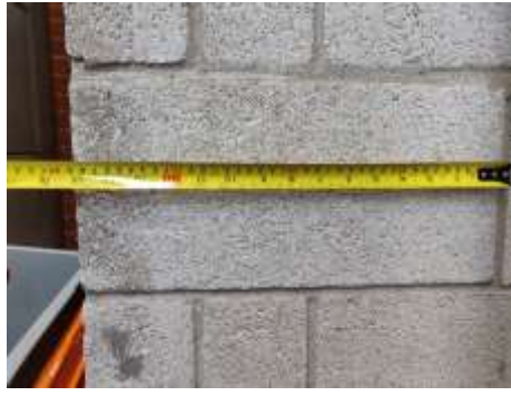
existing blockwork sizes
