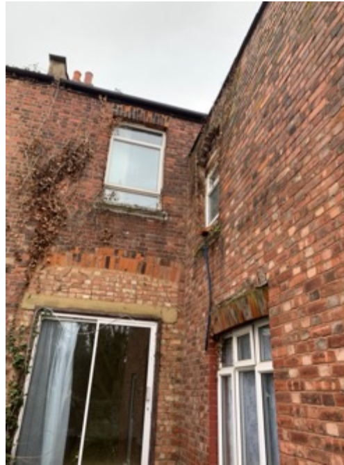
< Figure 01 – Rear brickwork failures
