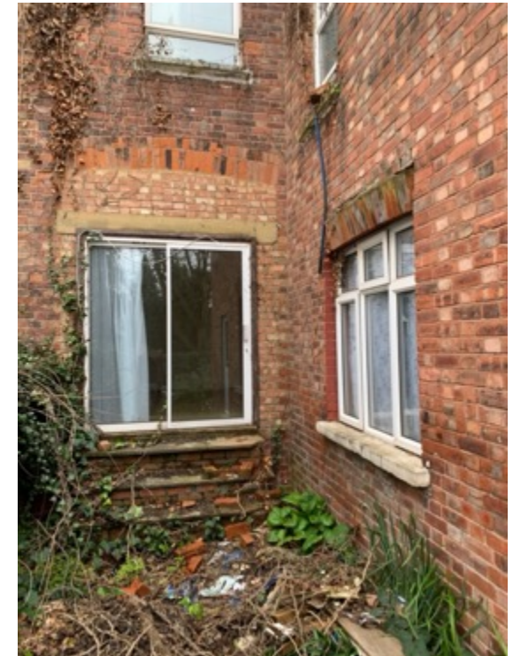
^ Figure 03 – Rear brickwork failures
