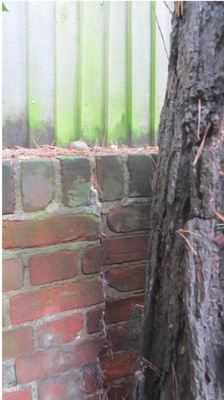
Photograph 3 - Showing the extreme proximity of the pine tree to the boundary wall with the wall displacement and cracking that it has caused
