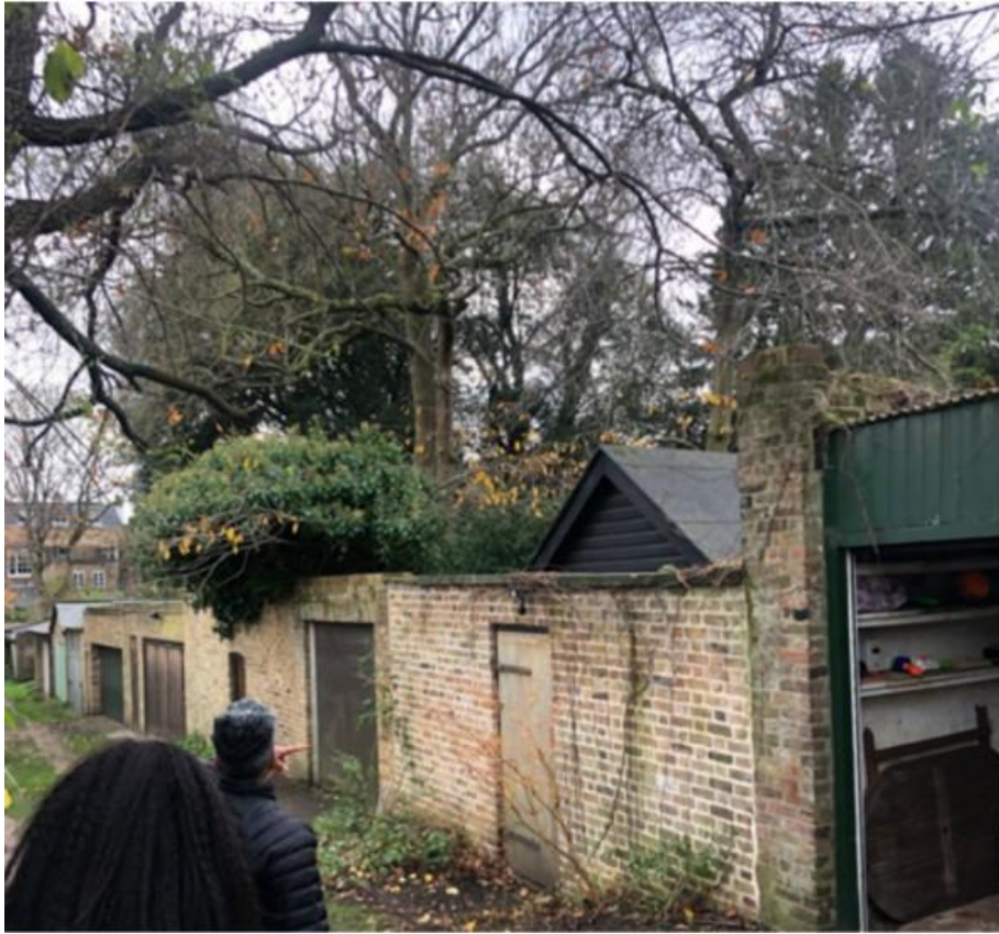
3. View of neighbouring garages from Grove Mews
