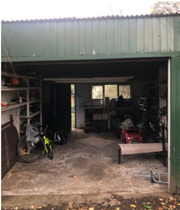
2. View of internal area
