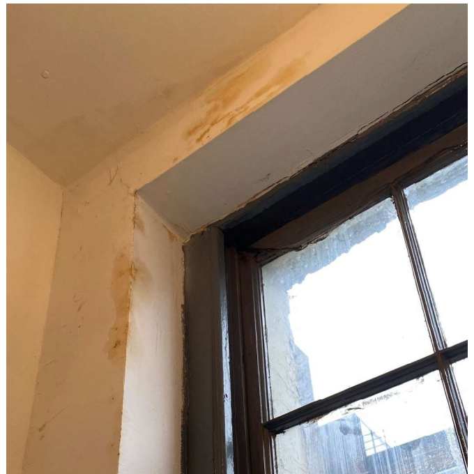
5.04 Water ingress around the staircase's window
