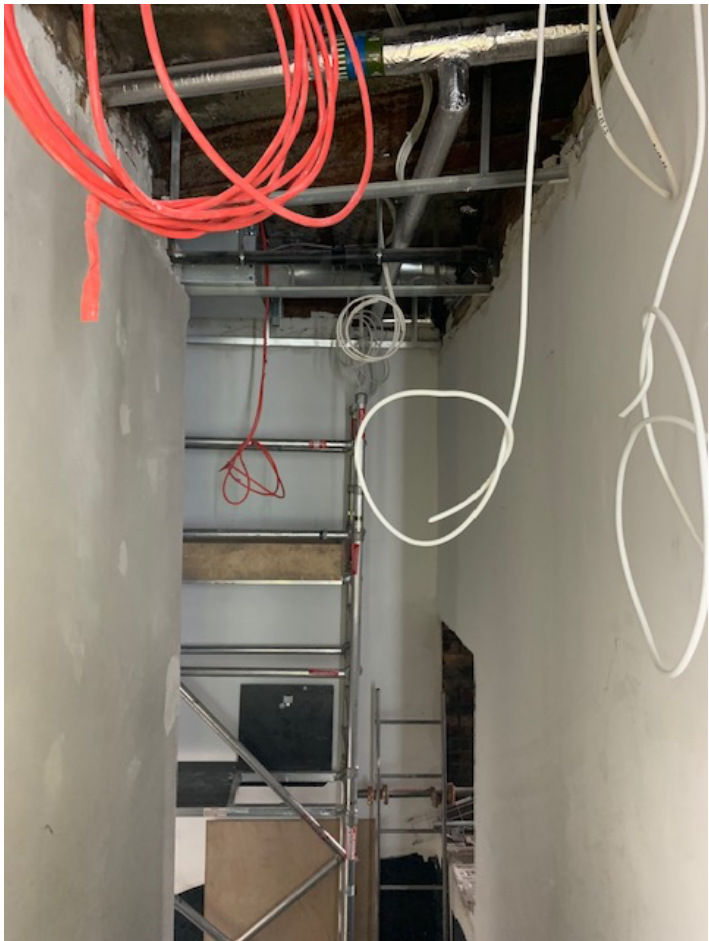
Proposed Metal Frame tight against services
