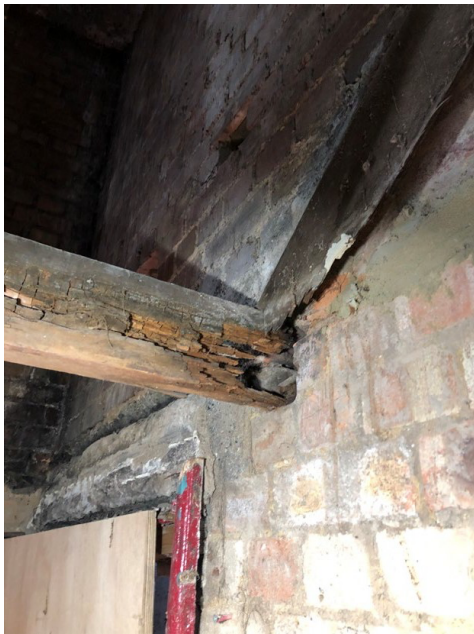
Rotten damaged timber frame
