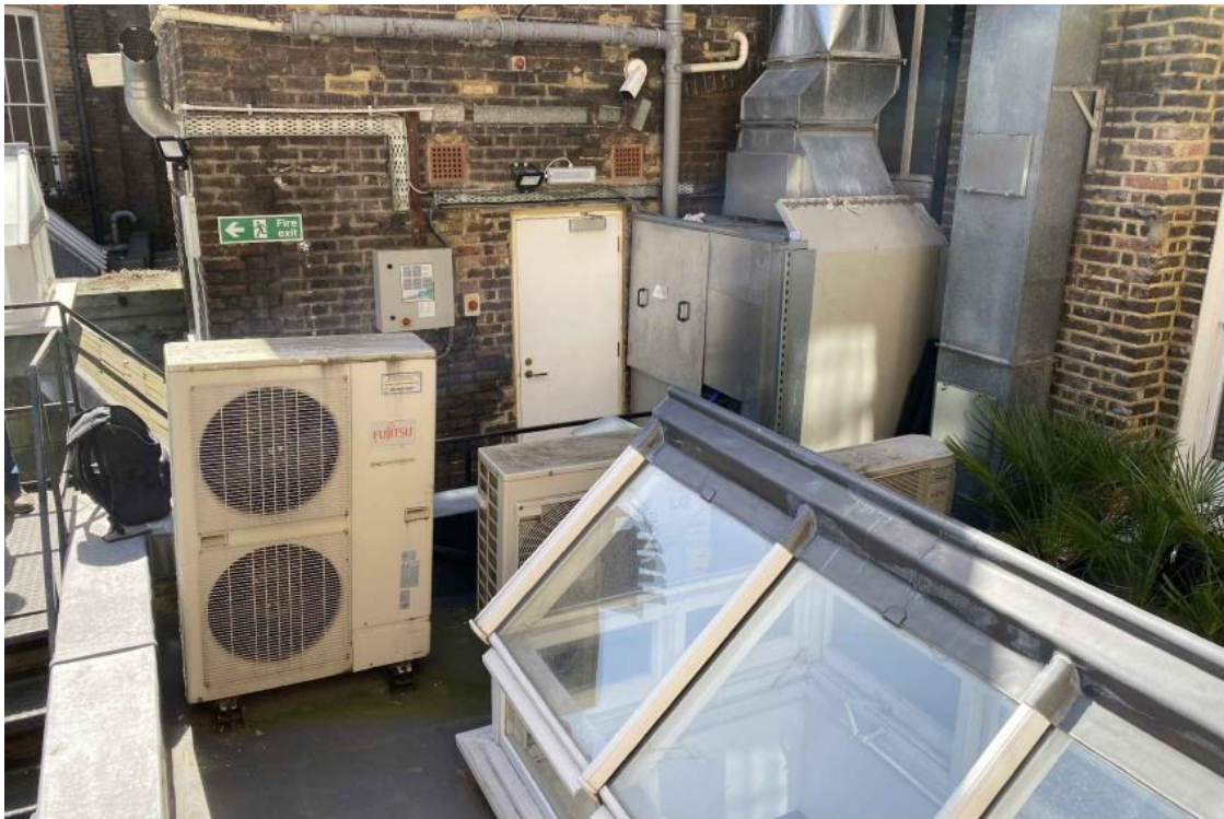
5. Application site roof looking on to rear of 8 Charlotte Street
