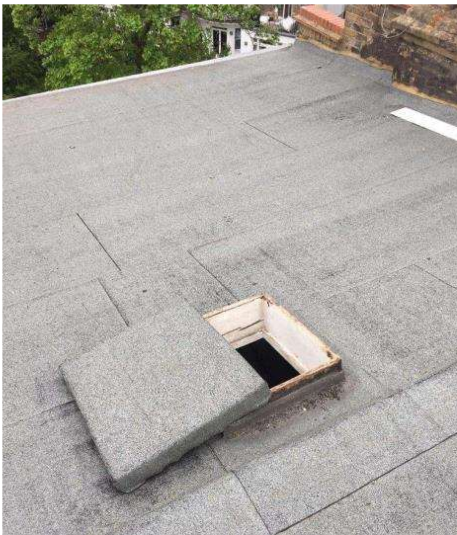
Photo 14 – Existing solid hatch to flat roof
