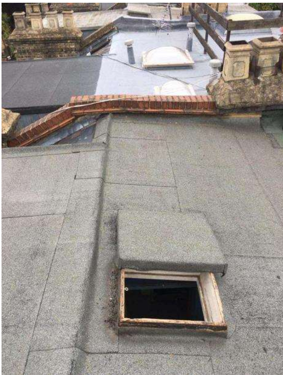
Photo 13 – Existing solid hatch to flat roof
