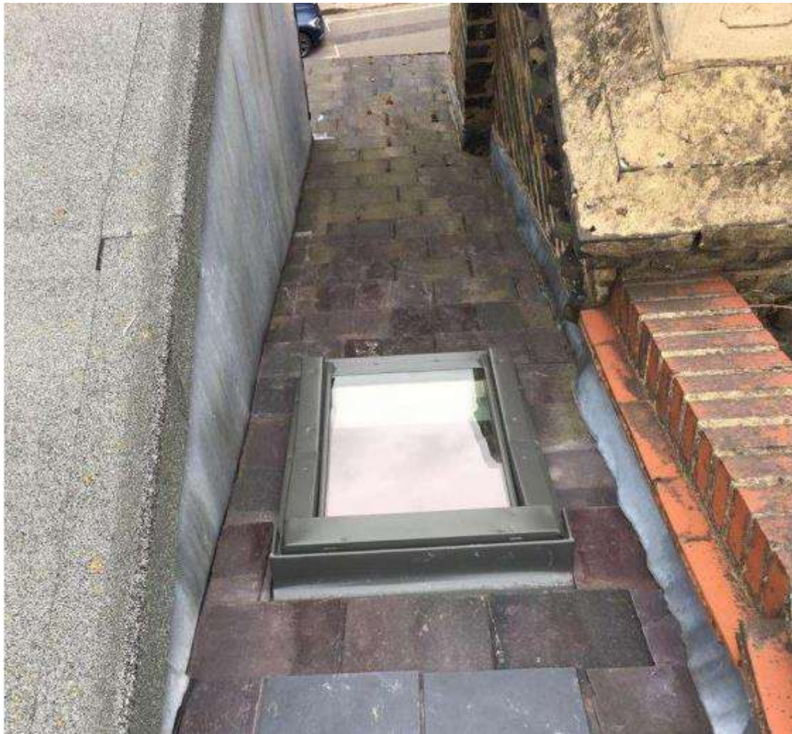
Photo 9 – Rooflight already in place (retrospective) to front roofslope in between dormer to the left and party wall/chimneys to the right.
