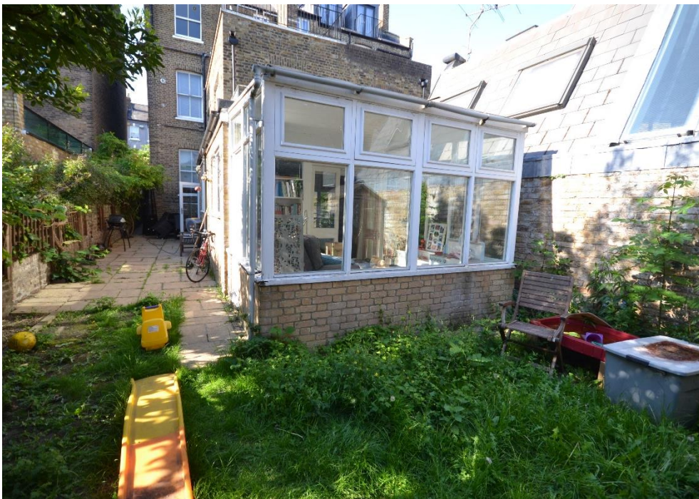
Rear view of No. 89.
