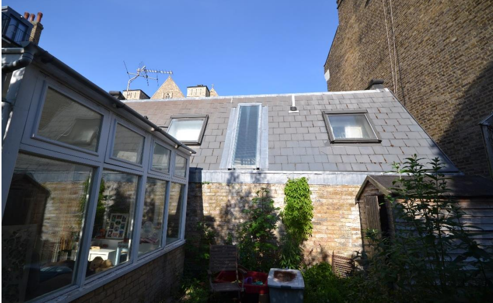
Side elevation of No.57 Shirlock Road.
