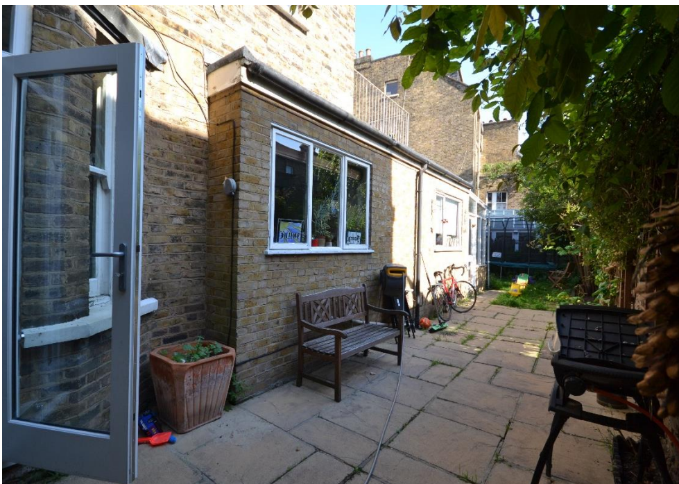
Side of existing ground floor flat existing extension and conservatory.
