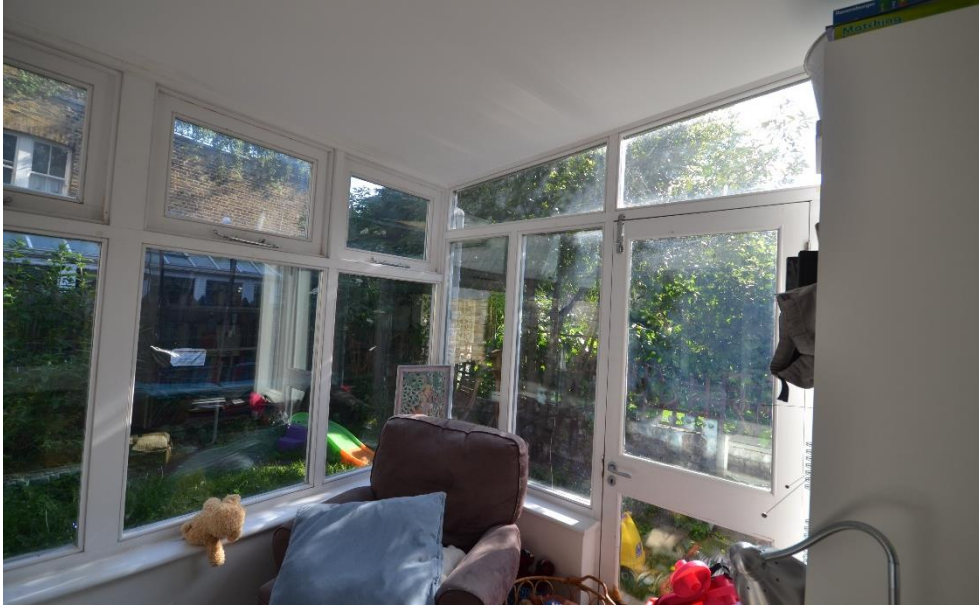
Inside of existing conservatory.
