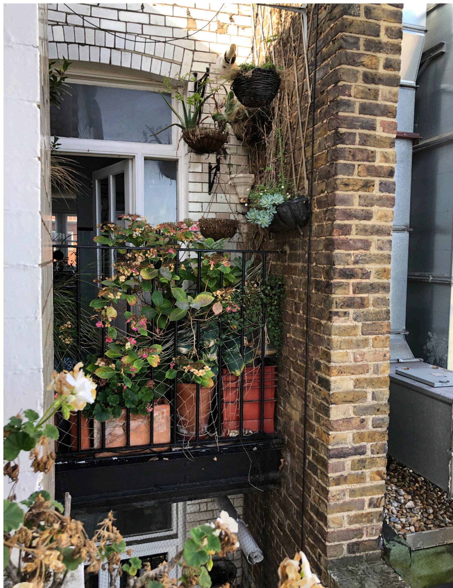
Existing: View of 4th Floor Balcony from flat window
