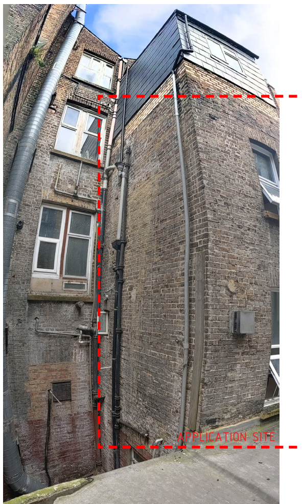
Rear View of 58a Belsize Lane
