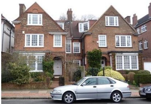
Nos. 40-42 Ferncroft Avenue
