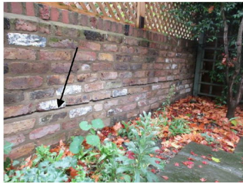
Cracking to rear left hand boundary wall
