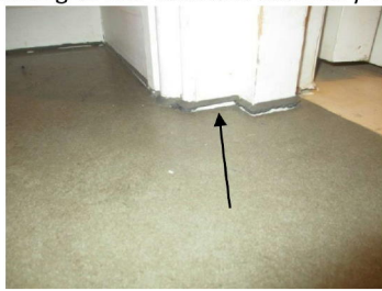
Cracking to rear left hand boundary wall
