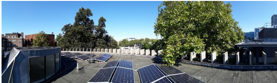
Figure B1: Measurement position on top of roof
