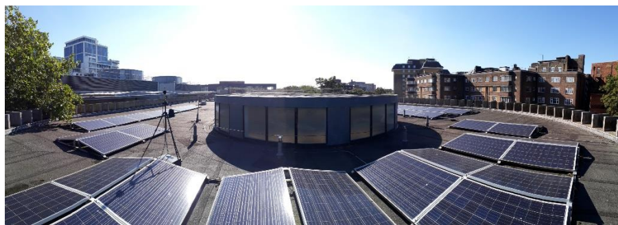
Figure B2: Measurement position on top of roof
