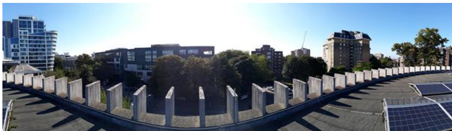
Figure B4: General view of surroundings from roof top
