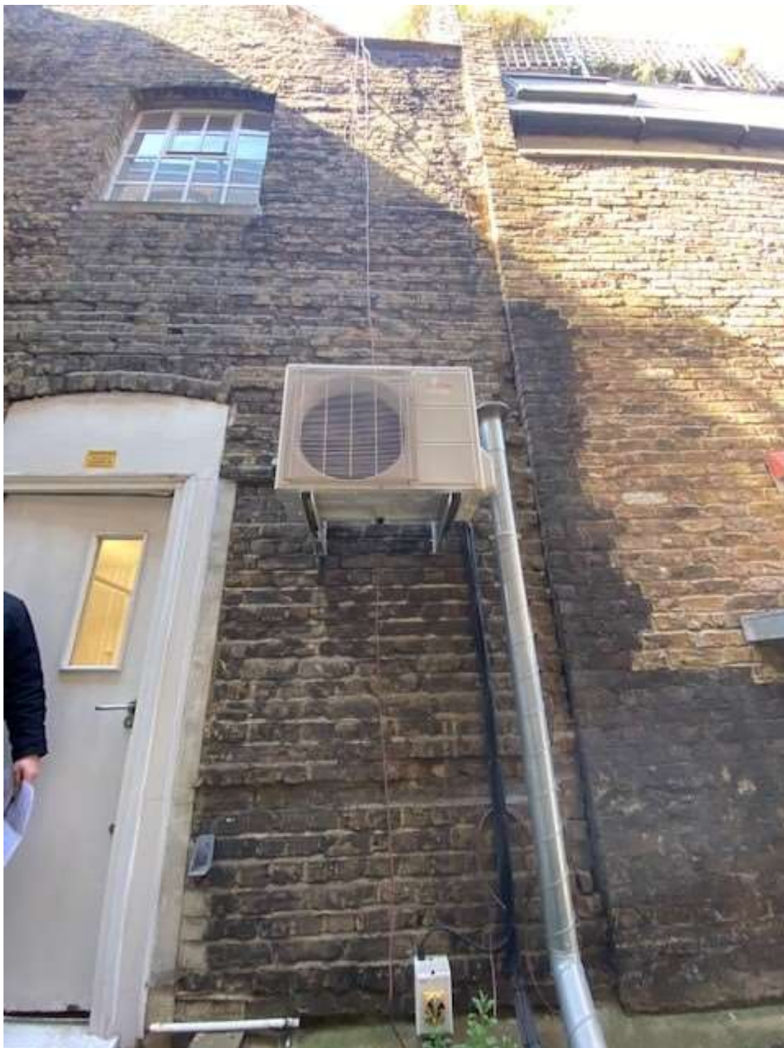
Photograph 2: The rear elevation where the new ducting is proposed
