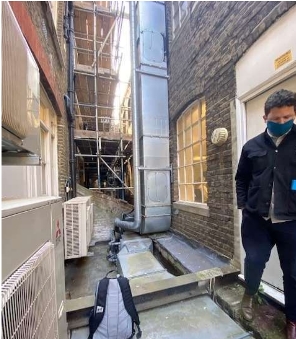
Photograph 3: The rear lightwell area showing existing lawful plant and ducting
