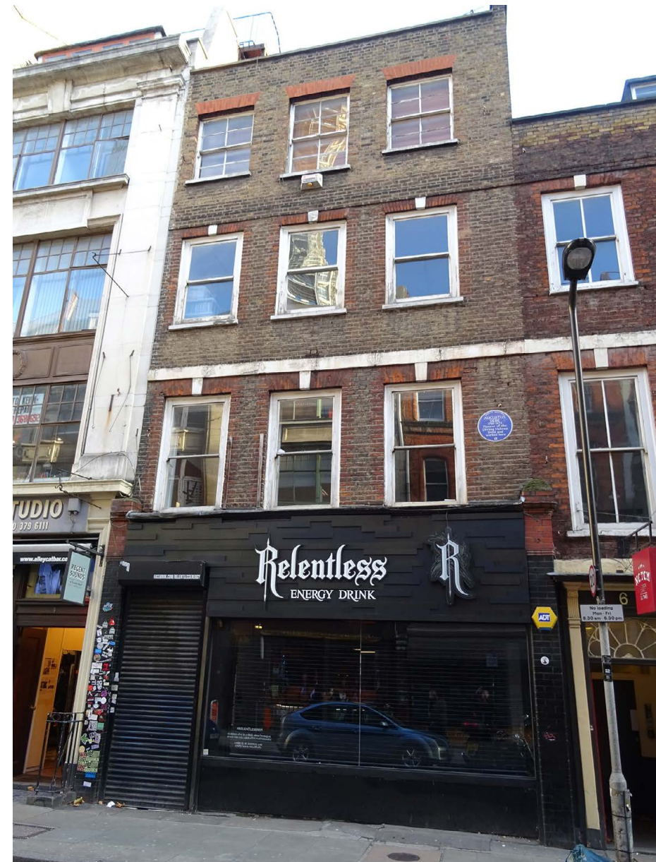
Fig. 1: Front elevation of No.5 Denmark Street
