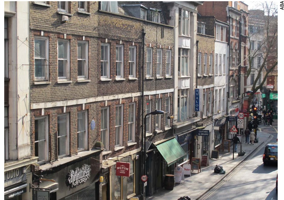
Fig. 20: General view of the south side of Denmark Street looking west. No.5 is in the foreground
