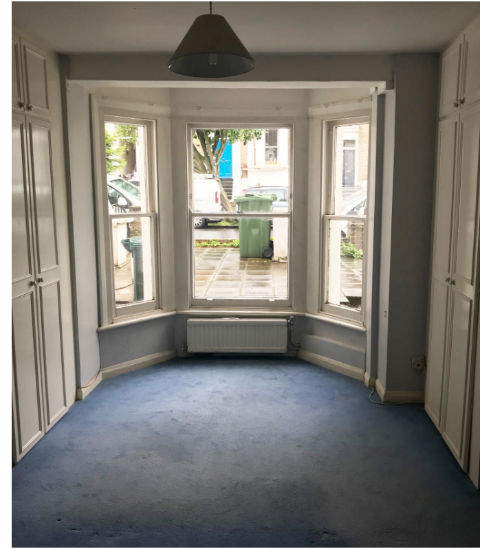
Internal view of lower ground floor bay window detailing to be replaced with double glazed versions to match the existing detailing.
