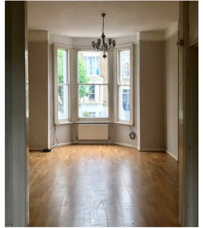
Internal view of upper ground floor bay window detailing to be replaced with double glazed versions to match existing.
