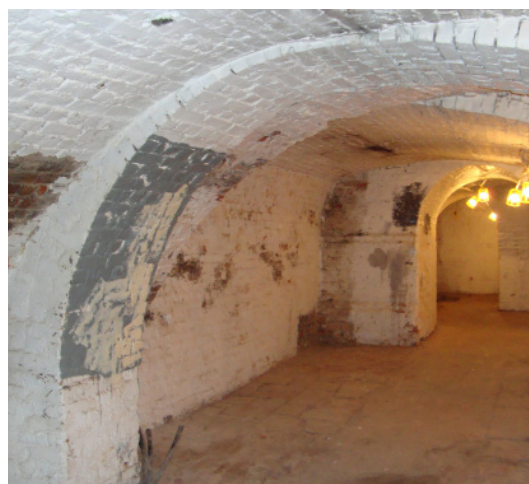
Convoluted damp walls prior to treatment.
