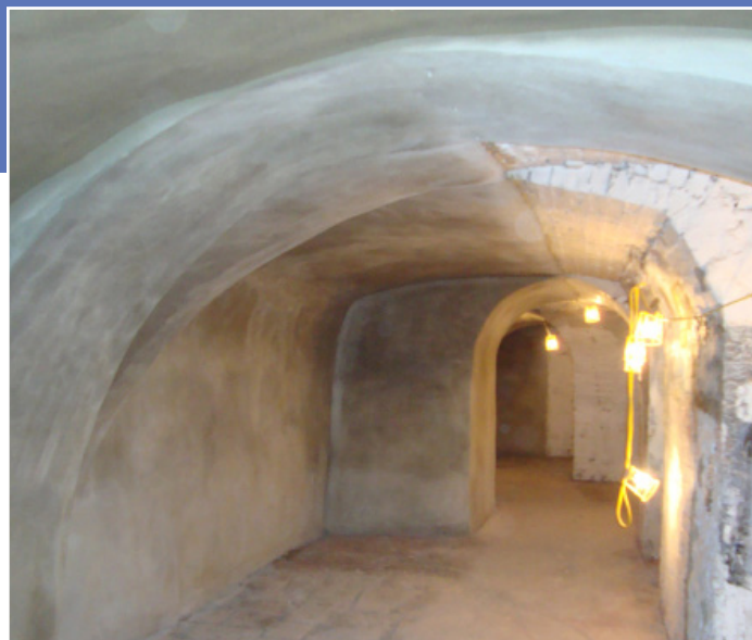
The surface ready for decoration, after two coats of Tarmac Whitewall.
