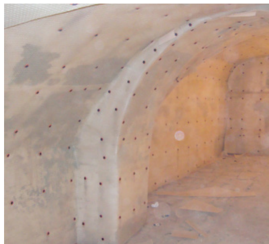
Application of Newton 508 mesh to vaulted areas.
